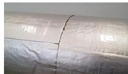
Step 12 Best results are achieved when overlaps are positioned one above, one below, one above configuration.
