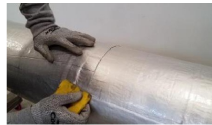
Step 3 Finish the butt strip using the spreader to ensure that the butt strip overlap is well adhered to itself and to the jacketing and without air bubbles.
