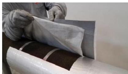
Step 10 Remove release film while applying jacketing around the circumference of the insulation. Apply pressure with plastic spreader to ensure that the butyl adhesive fills the surface cells of the insulation and achieves adhesion without trapping air.
