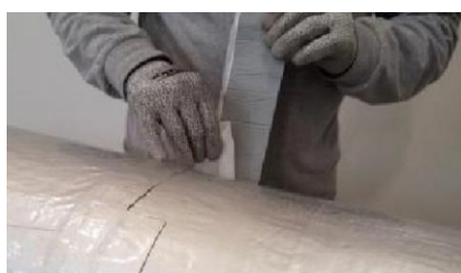
Step 2 Apply butt strip in the same way as the jacketing, peeling the release film away while wrapping the strip around the insulation.
