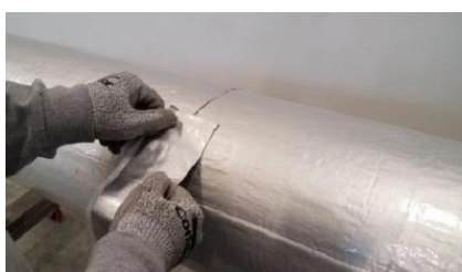
Step 1 If the insulation is supplied with pre-applied jacketing, then a circumferential butt strip will need to be applied to seal over the joint.
