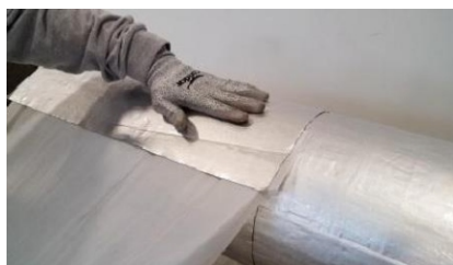
Step 11 Remove remaining release film and press jacketing around the circumference to achieve adhesion without trapping air.
